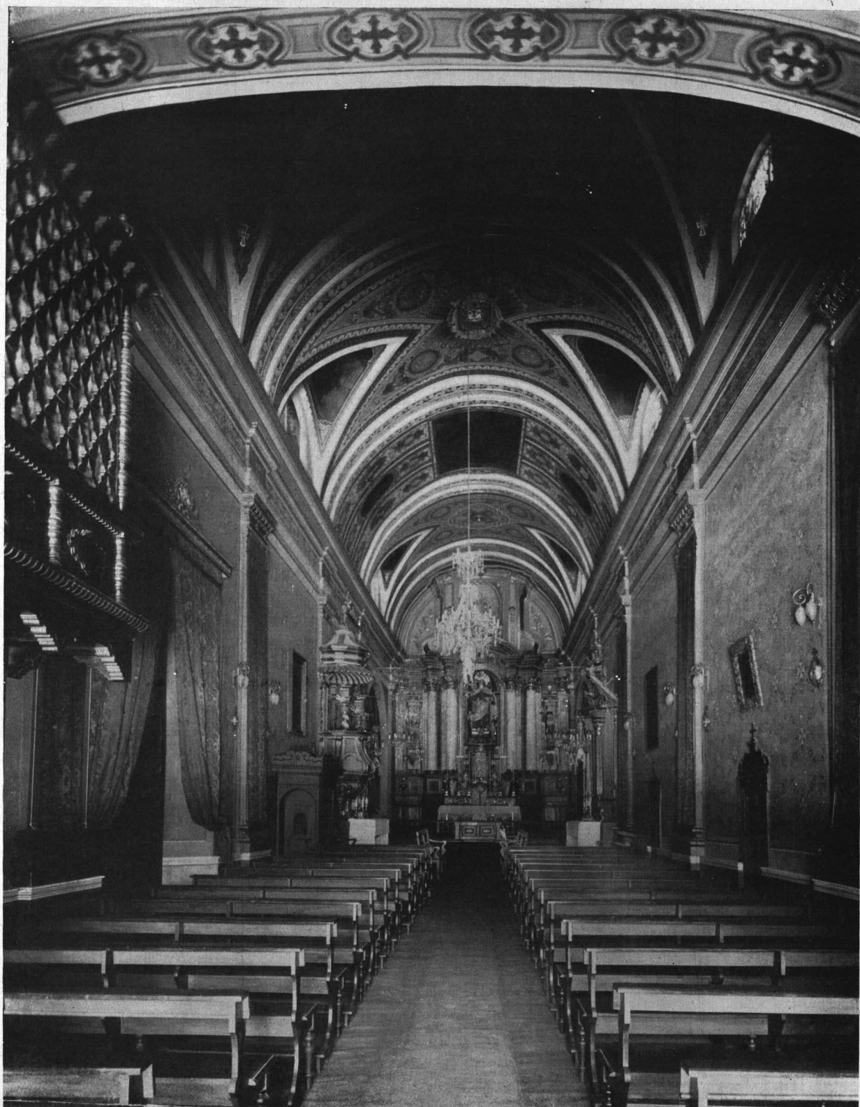
Vista general del interior
