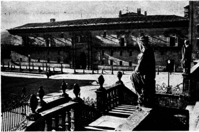
14. Santiago de Compostela, hospital real, fachada.
